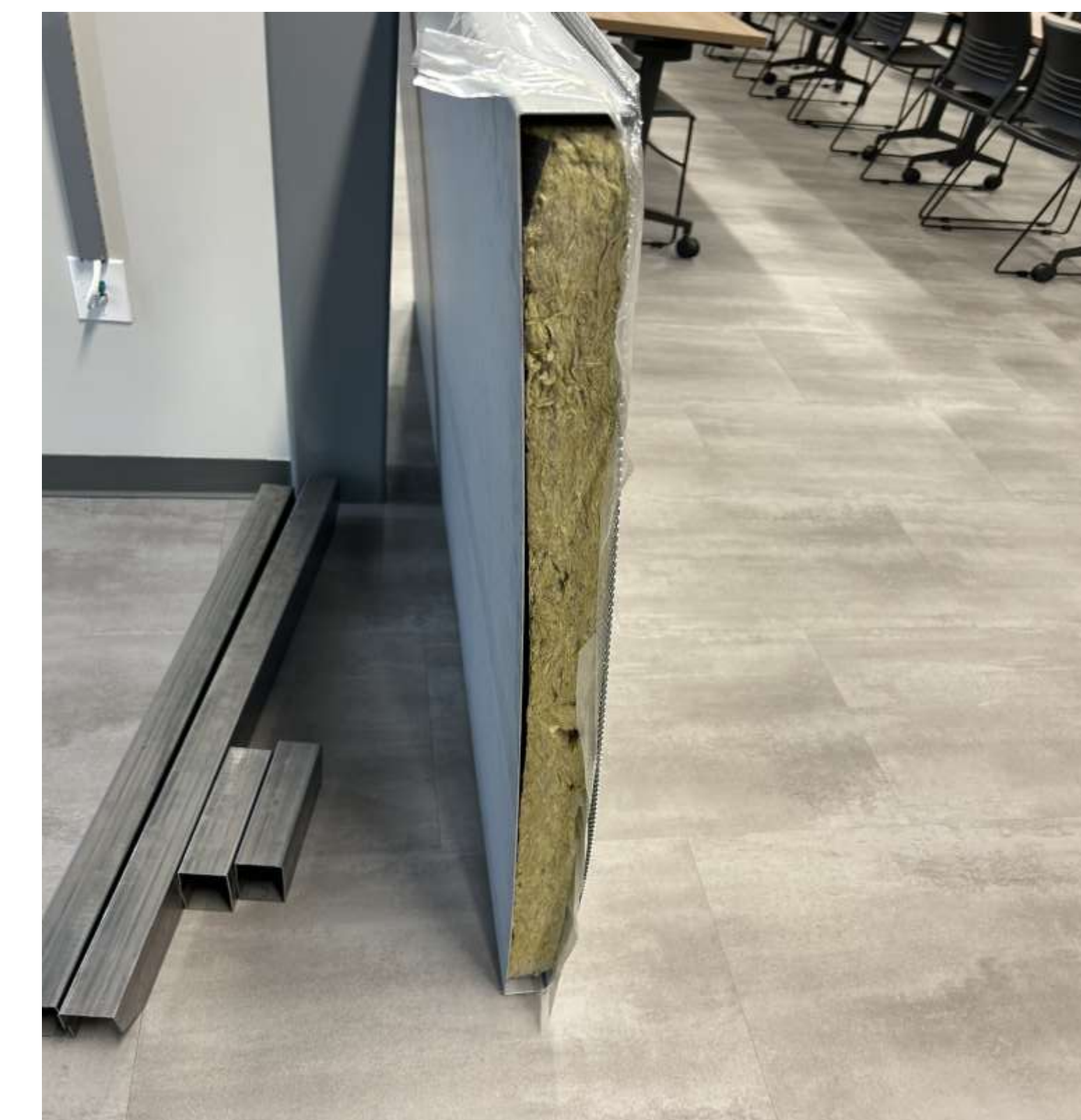
Figure 6: Cross-section view of sound panel (w/insulation)
