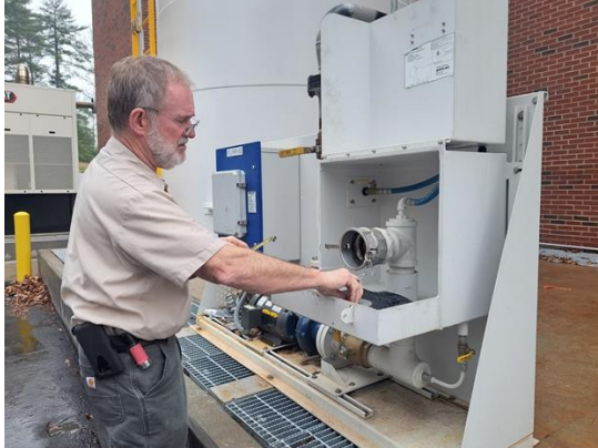
Preparing for fuel delivery at Steam Plant
