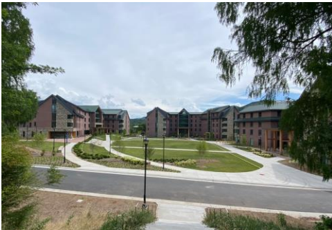
New Lower Campus Residence Halls (“Rocks”)
