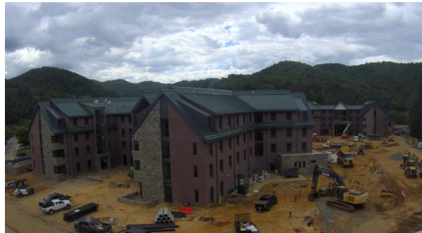
Construction of Lower Campus Residence Halls
