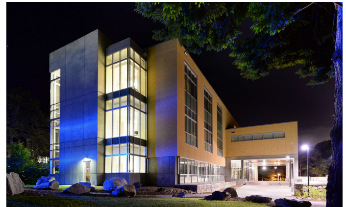
Above: UNC Asheville's Zeiss Science Building, a science and classroom facility constructed by Rentenbach.
