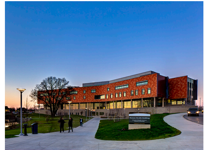
Above: The Human Health Building at Oakland University.
