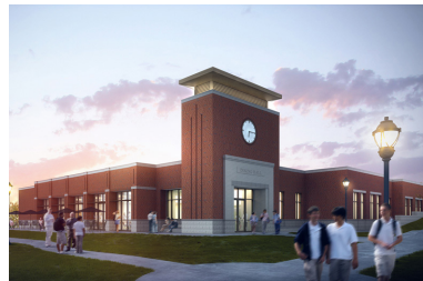
Tennessee School for the Deaf New High School and Dining Hall $20 million
