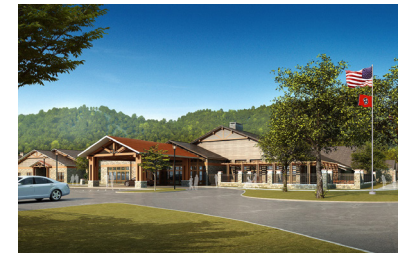
The State of Tennessee Cleveland, TN Veterans Home $31 million
