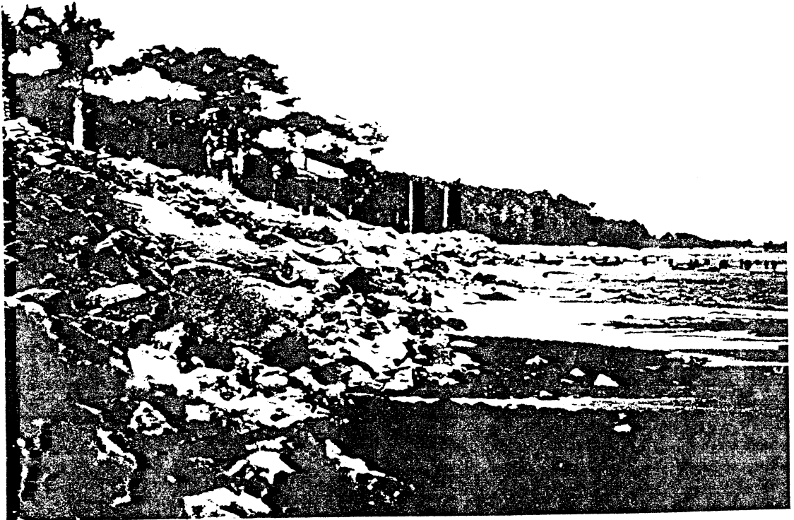
Figure 2. A view of the low tide beach at Sea Island, Georgia, demonstrating how this type of stabilization is unsightly, produces rubble making swimming dangerous, and reduces access to the beach. Clearly no high tide exists in front of this wall.
