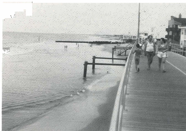
Figure 3. A scene on the Ocean City, New Jersey shore, site of one of the least successful replenishment projects. A $5 million plus beach disappeared in 1982 in 2.5 months.
