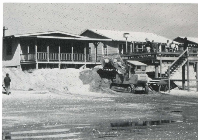
Figure 5. A poor man's replenishment technique. Here a bulldozer moves sand from the low tide beach to the upper beach on Topsail Island, North Carolina. The family owning the beach cottage looks on with high hopes. The bulldozed pile of sand disappeared in the next minor storm.
