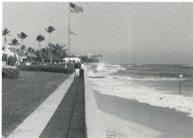
Figure 1. Shoreline erosion on beachless Palm Beach, Florida. Here a combination of natural shoreline retreat and acceleration of surf zone processes caused by the seawall has taken away the beach. The community values buildings over the beaches.
