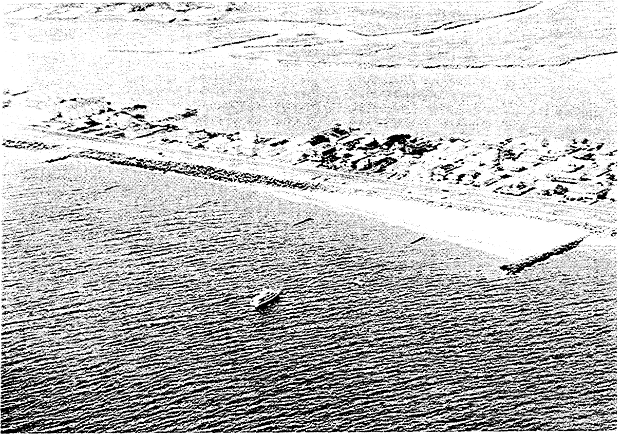
Figure 8. A seawalled section of the coast where the dry beach exists only on the updrift side of groins. Most of the New Jersey coast that has shore parallel structures also has a groin field as seen in this photograph of Sea Bright.
