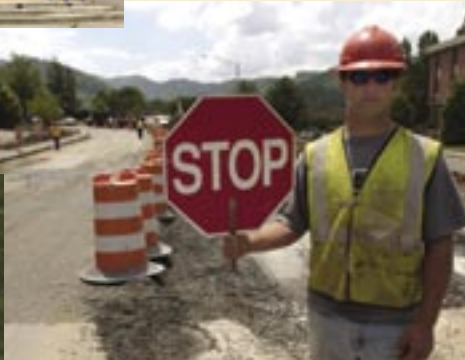
Centennial Drive Project
