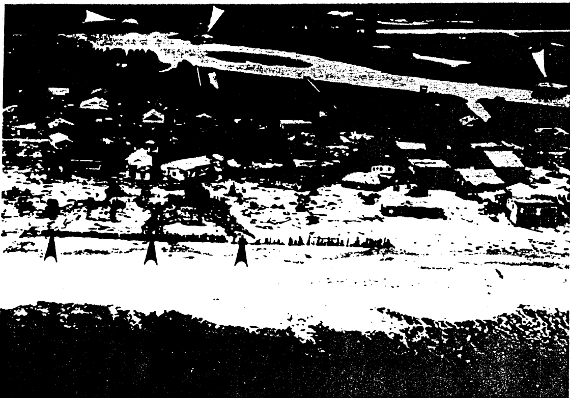
Figure 12. On Pawleys Island, storm surge ebb channels (black arrows) were incised well into the island, frequently cutting through bulkheads, causing their ultimate failure in a seaward direction. The photo also shows an excellent example of what we defined as "new gap," where beachfront buildings were destroyed and/or removed from their foundations. Note also the three houses carried by storm surge into the backbarrier marsh (white arrows).
