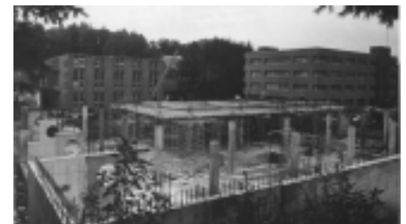
New Addition Construction
