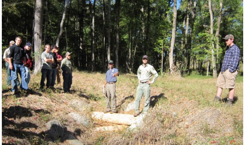
Examining stream restoration structures at Hunting Creek.
